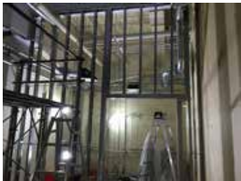
Partition wall construction
