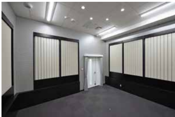
Installation example of water-cooled radiant panel system
