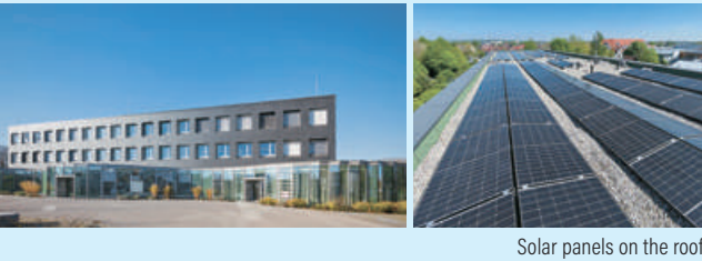
Solar panels on the roof
